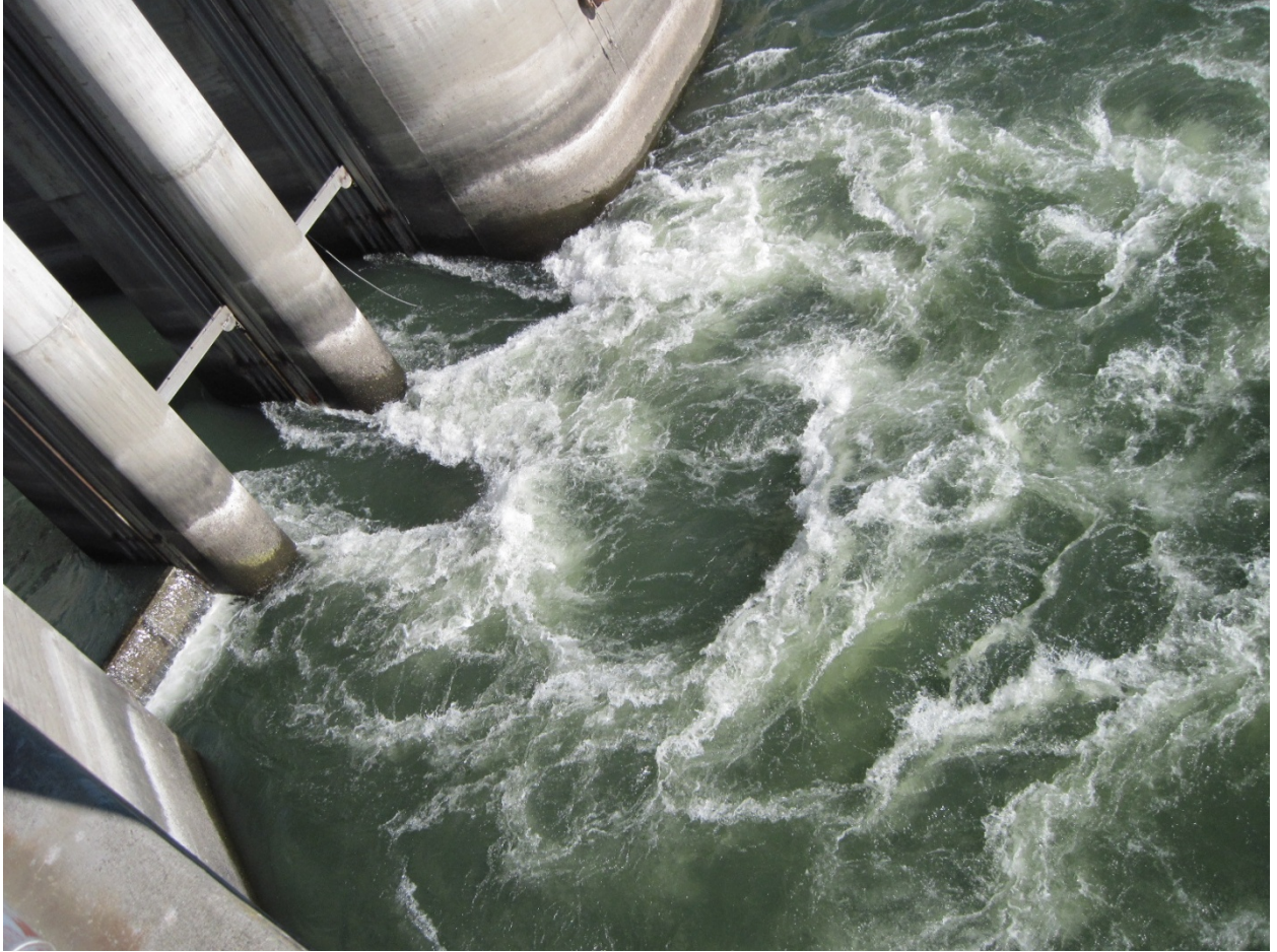
Figure 1 - East entrance 2.0 ft differential, 8.5 ft gate open
