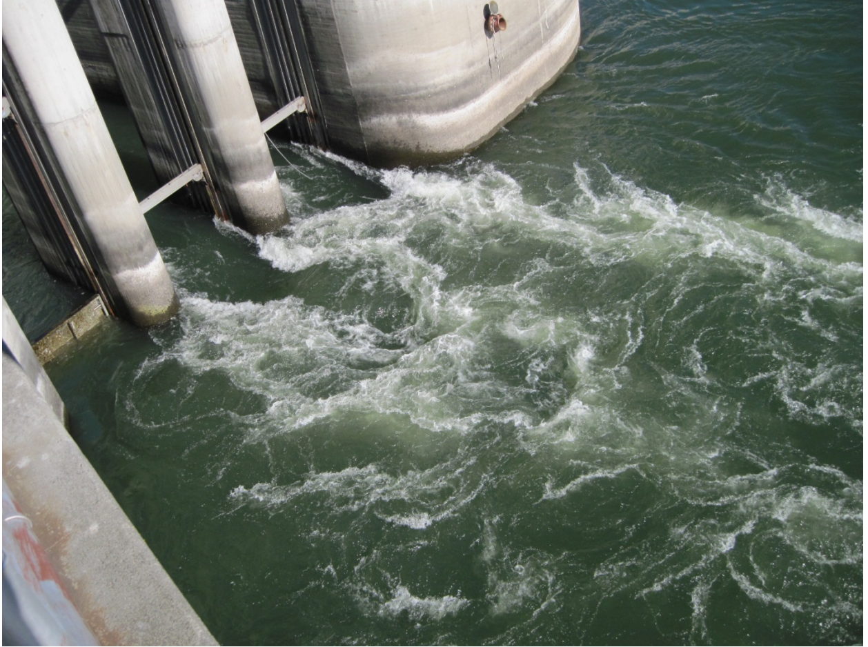
Figure 2 - East entrance 1.5 ft differential, 10.7 ft gate open
